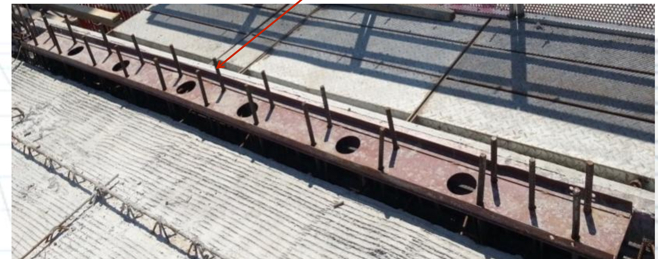
Steel bar position inspection template
